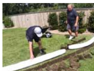
1. Position QuickDrain
