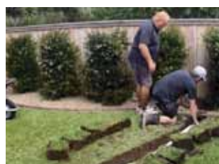
3. Lay QuickDrain
