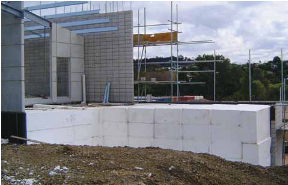
EXPOL GeoFoam as lightweight fill under a concrete floor
